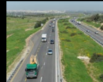
Highway 6, Cross-Israel Highway
