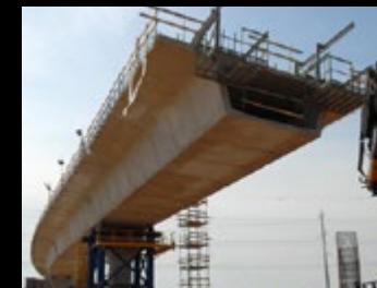
Segment bridge up to 66-meter span
