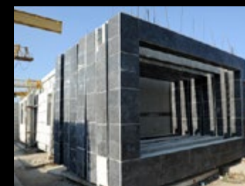
Exterior walls, granite cladding
