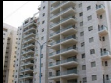
Naveh Towers, Rehovot Apartments: 163 Total of 28,810 sq.m.
