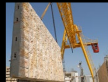
Lifting a retaining wall element
