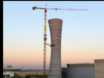
Control Tower, Ben Gurion Airport Total of 8,000 sq.m.
