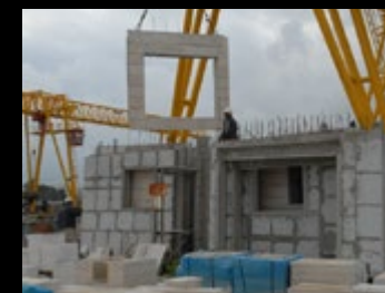
Lifting an exterior wall
