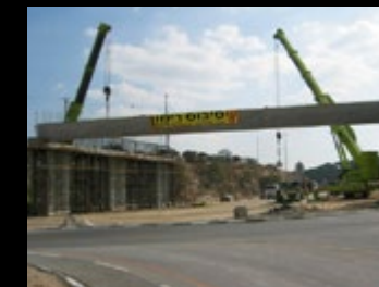
Assembling channel cross-section bridge beams
