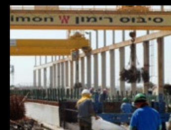
Production line: prestressed beams, beams for industrial structure
