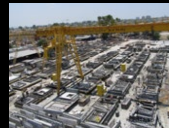
Production line, exterior walls
