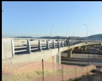
722 Railway Overpass, Yokneam
